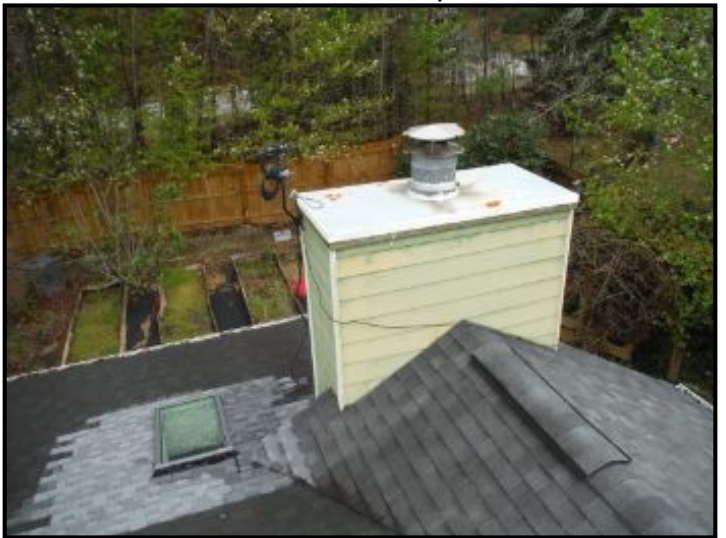
View of roof and chimney.
