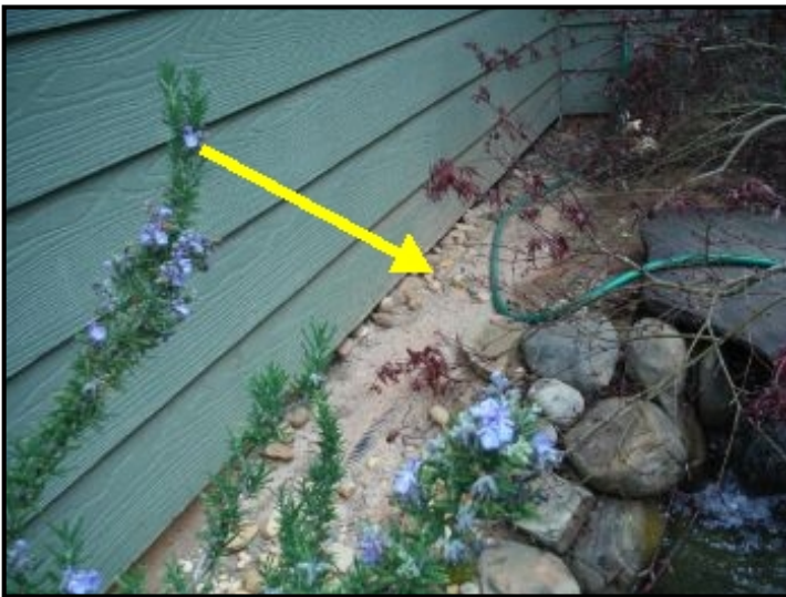
Remove soil at garage wall to
