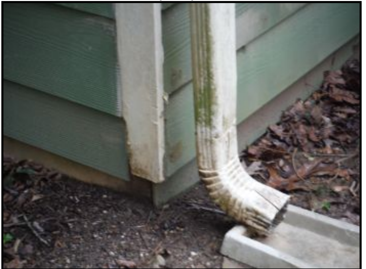
Secure the downspout to the exterior wall on left rear corner.
