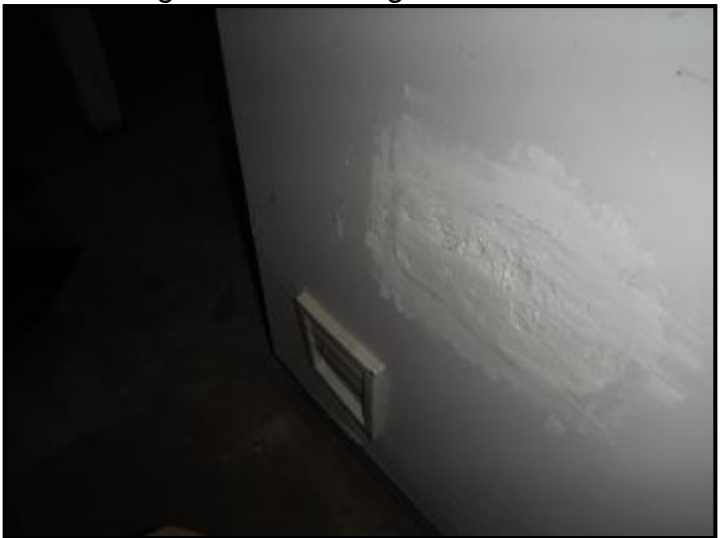
Dryer vent in garage.
