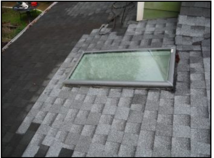
View of roof over rear porch area.
