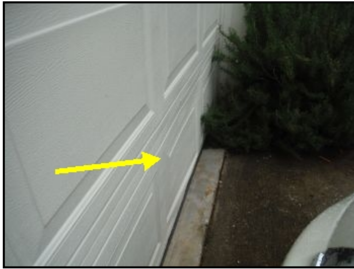
Slight dent in garage door.
