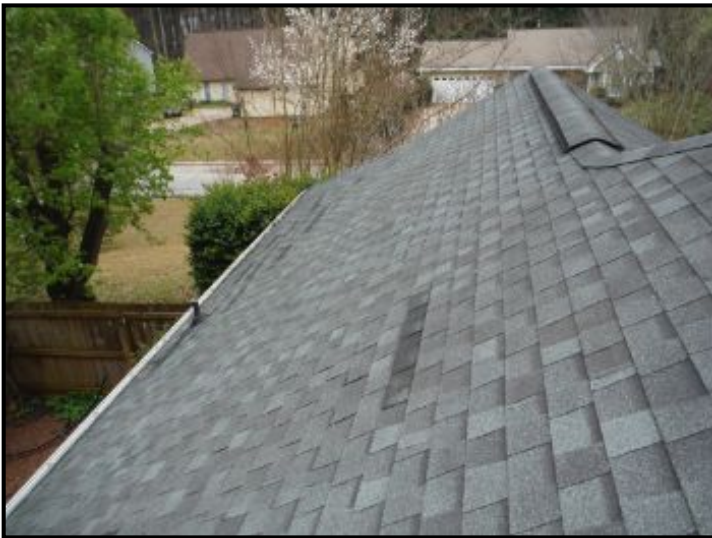
View of roof
