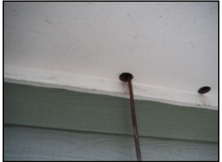
Seal holes in soffit above the water heater.
