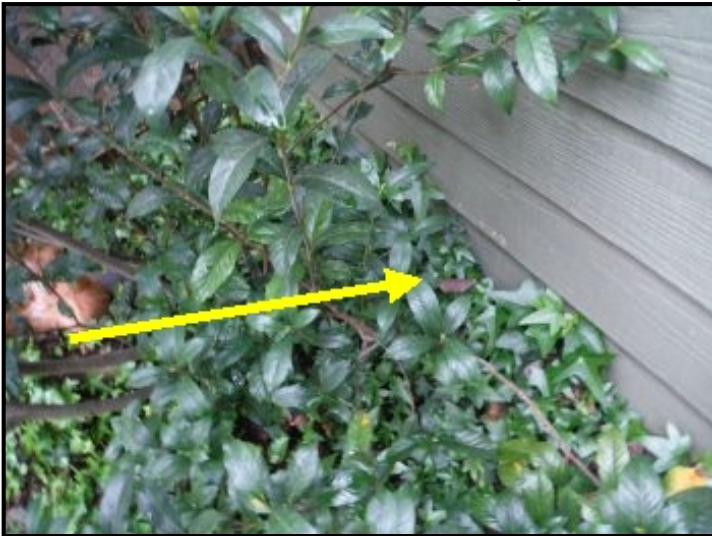
Remove ground cover to expose foundation.
