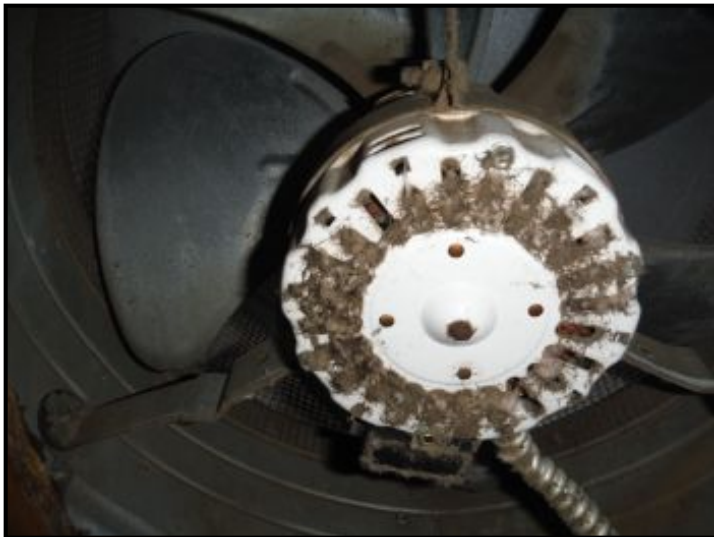
Clean the vent fan in attic.
